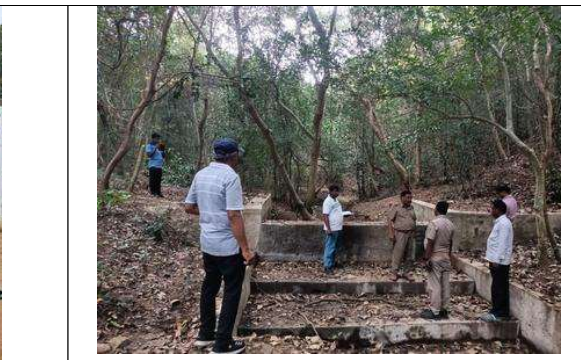
Check Dam (SMC Work 2022-23)
