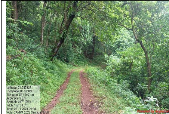
Forest Road Repair, Similipal South Div.
